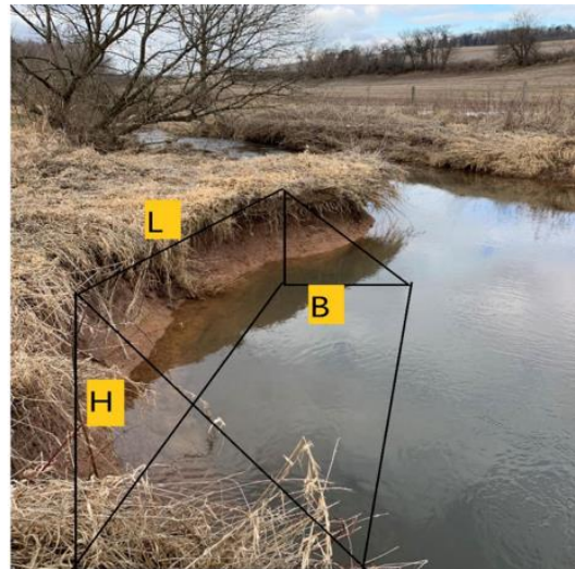
Figure 1a: Before bank reinforcement (source: PA F&BC)
