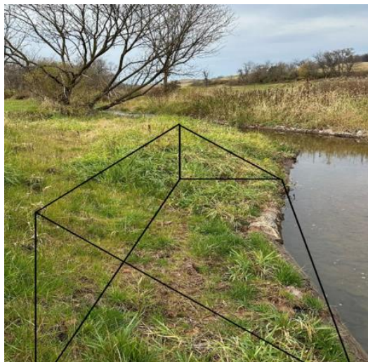
Figure 1b: After bank reinforcement (source: PA F&BC)
